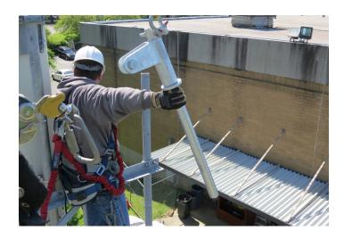
Antenna mast pipe, attachment points to the boom, and boom attachments must be inspected prior to installation of the Lite Gin Pole to ensure all connectins are up to relevant standards.
